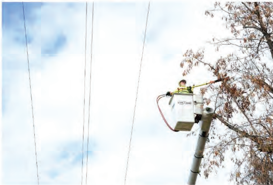
Figure 4 A contractor trims trees in a bucket truck
