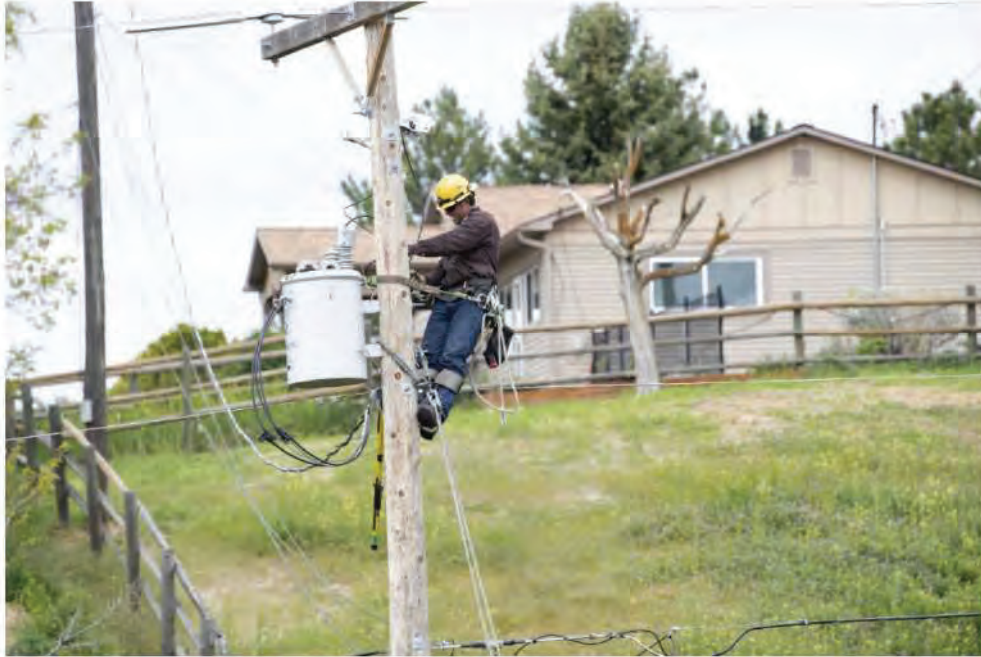
Figure 2 A line worker installs a spark prevention unit near Eagle, Idaho
