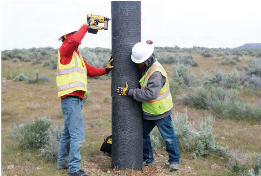
Figure 1 A field team installs a mesh wrap on a wood pole in 2022
